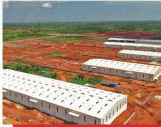
Warehousing Complex Benin
