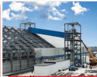
Urea Bulk Warehouse & Conveyor Nigeria
