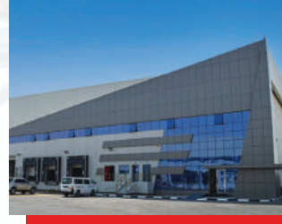
Logistics Centre United Arab Emirates
