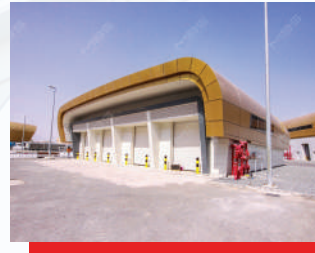
Dubai Metro Depo Dubai
