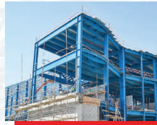
Logistics Centre United Arab Emirates
