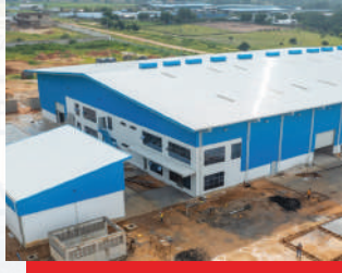
Pipe Factory Tanzania
