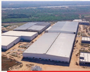
Automobile Production Facility Pakistan
